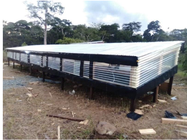
Construction of modern solar dryer
