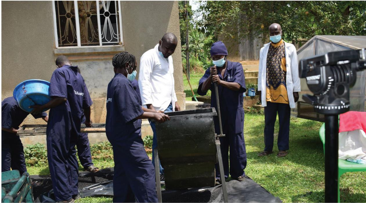
*Figure 1 Crushing of charcoal dust to fine particles to easy production of briquettes*
